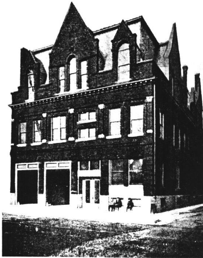
Early view of City Hall and Fire Department Building built in 1908 under the direction of C.C. West of the Borough Council. The divided doorway to the bays of the fire department were eliminated about 1930 to accommodate changing needs as were the manure pit and hayloft formerly located at the rear of the building.
