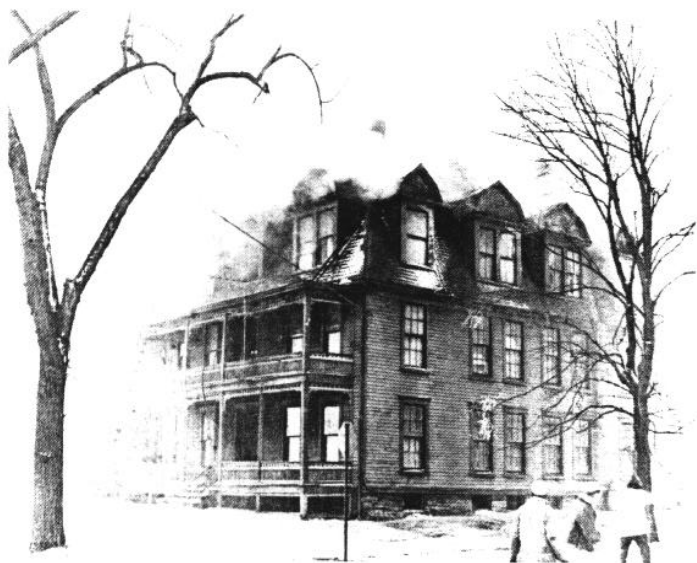
The Burdick Block at N. Lehigh Ave. and Allison St. burned in January of 1963.
